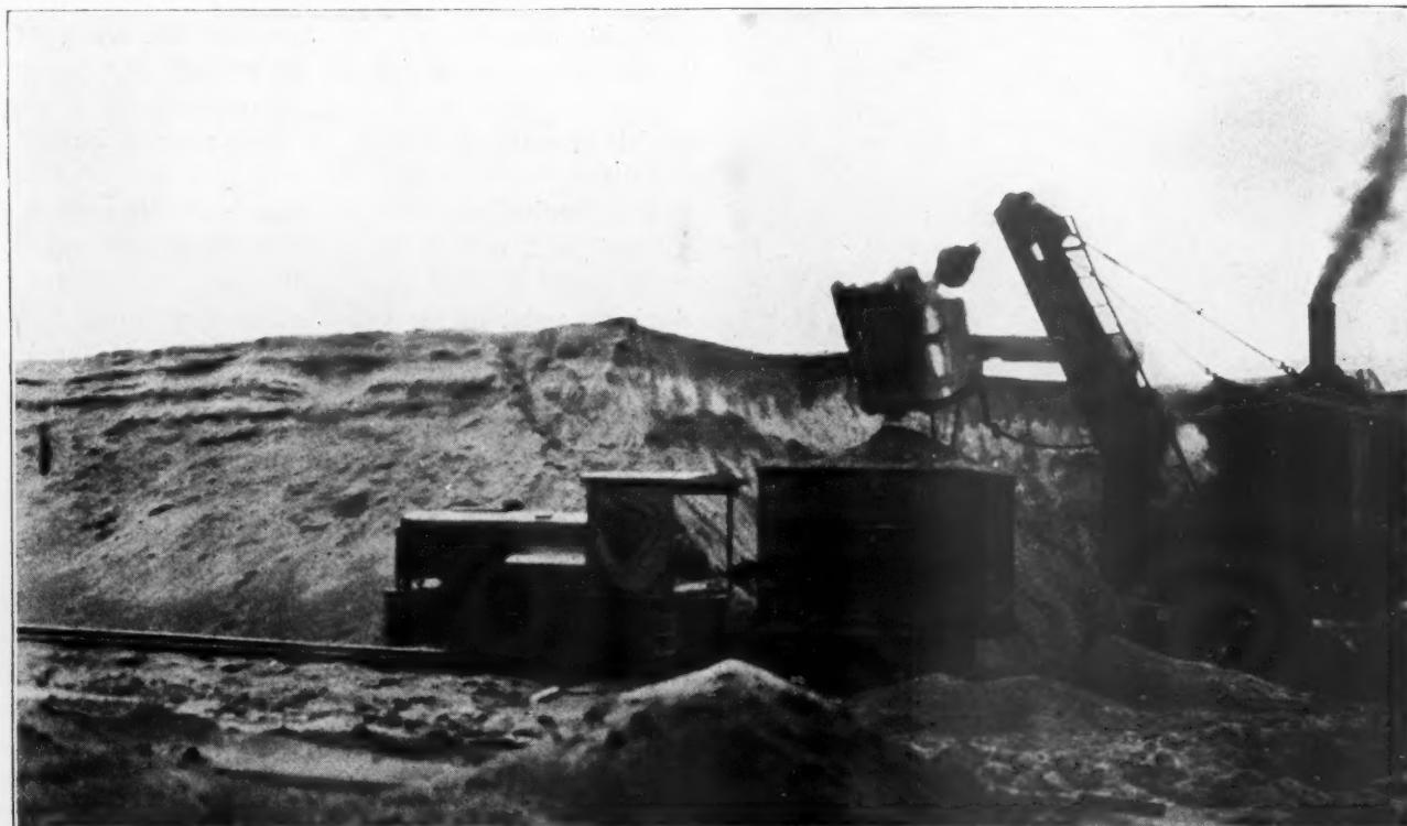
Excavating at the Bank and Loading Sand Cars
